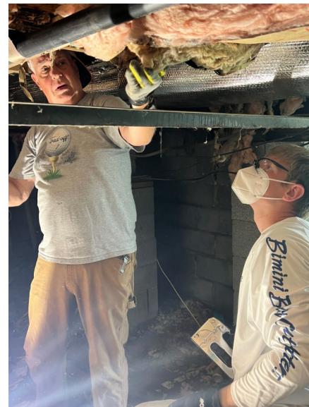
Tom and Toby insulating the bathroom floor
